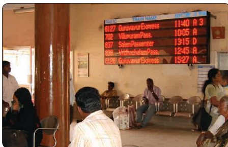
5 Line Display Installed at Vriddhachalam Jn. Railway Station (Chennai)
