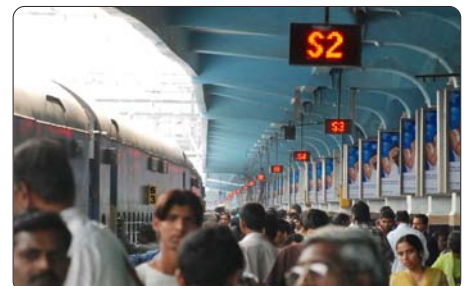
Coach Guidance Installed at Secunderabad Railway Station
