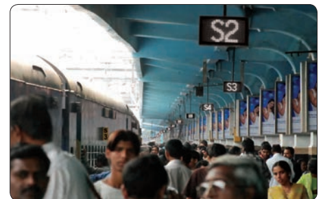
Coach Guidance Installed at Secunderabad Railway Station
