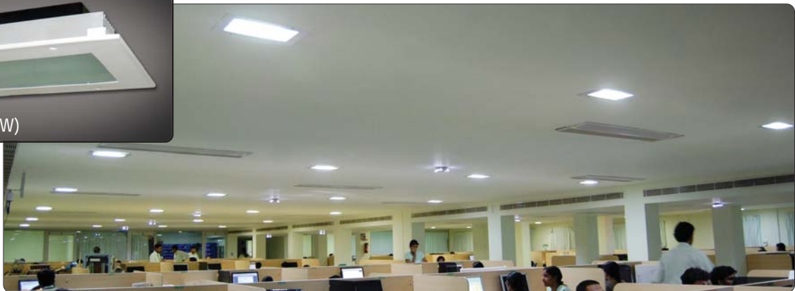
Room Size: 160 X 65feet 56W X 60 Nos ( 3360W ) Fluorescent Luminaire Replaced with 14W X 48 Nos ( 672W ) LED Luminaire
