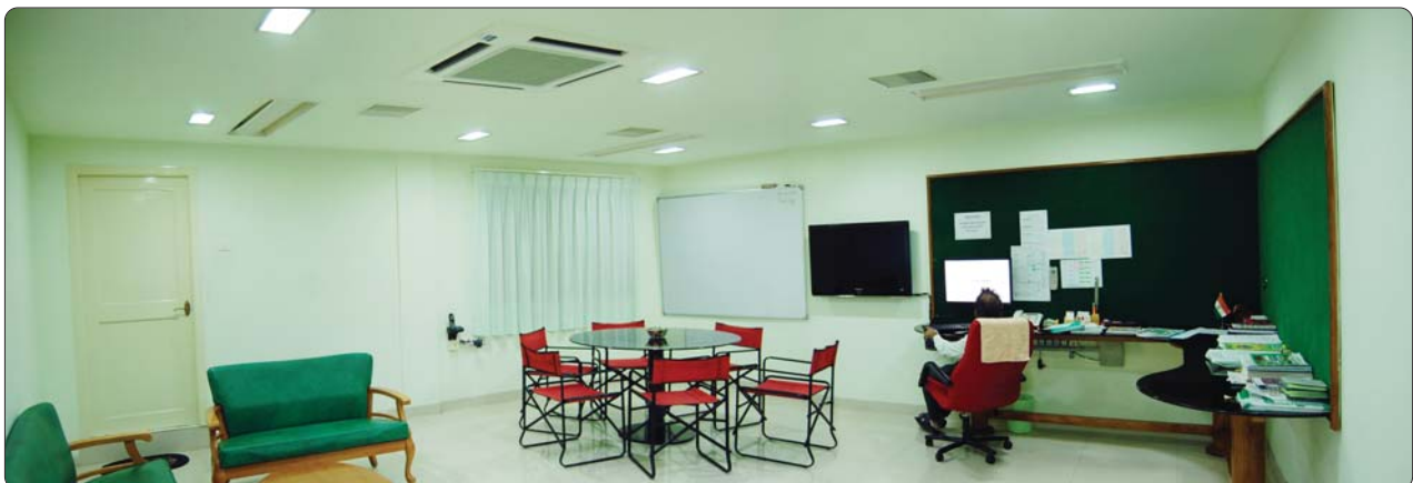
Room Size: 18 X 20feet 56W X 8 Nos ( 448W ) Fluorescent Luminaire Replaced with 14W X 9 Nos ( 126W ) LED Luminaire.
